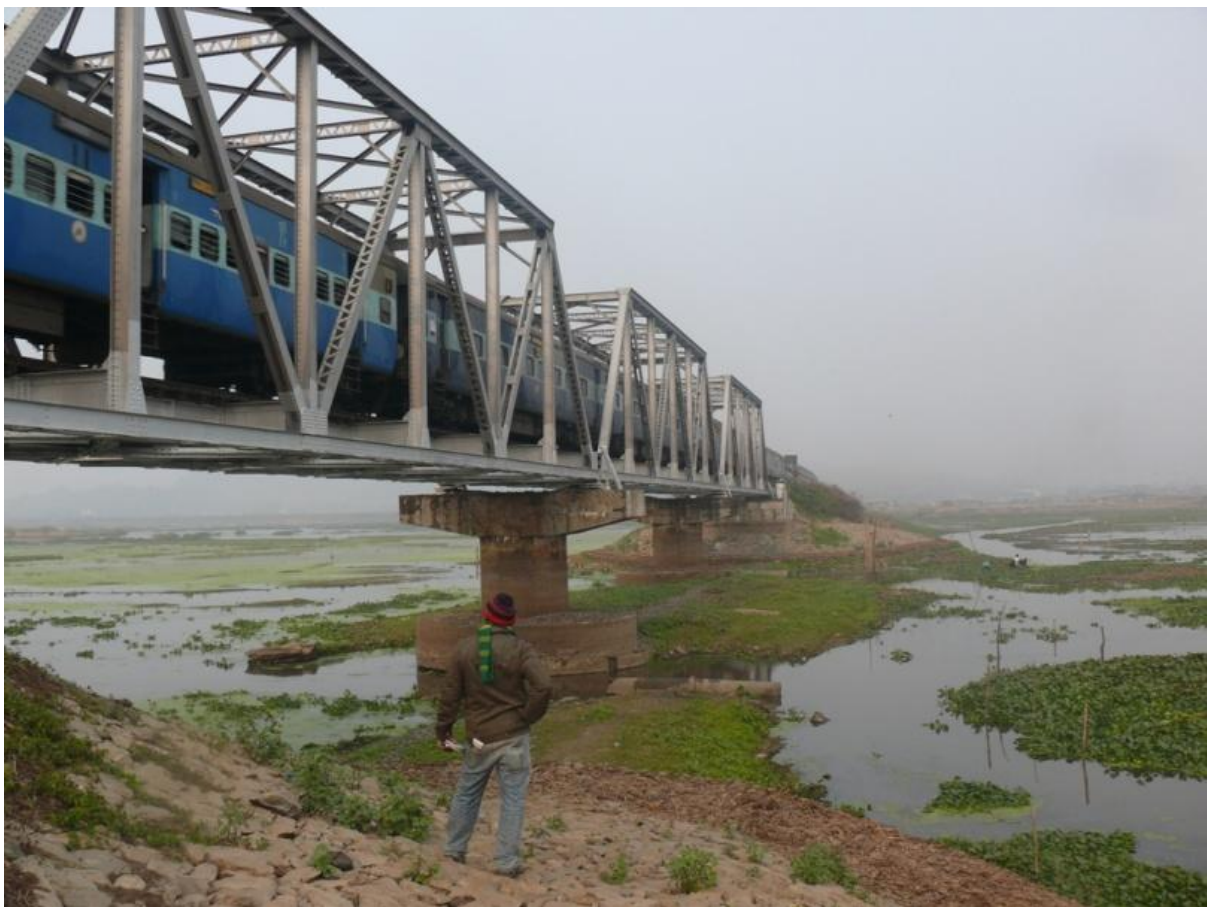
Photo 12: The Railway track passing through the southern part of the Deepor Beel
