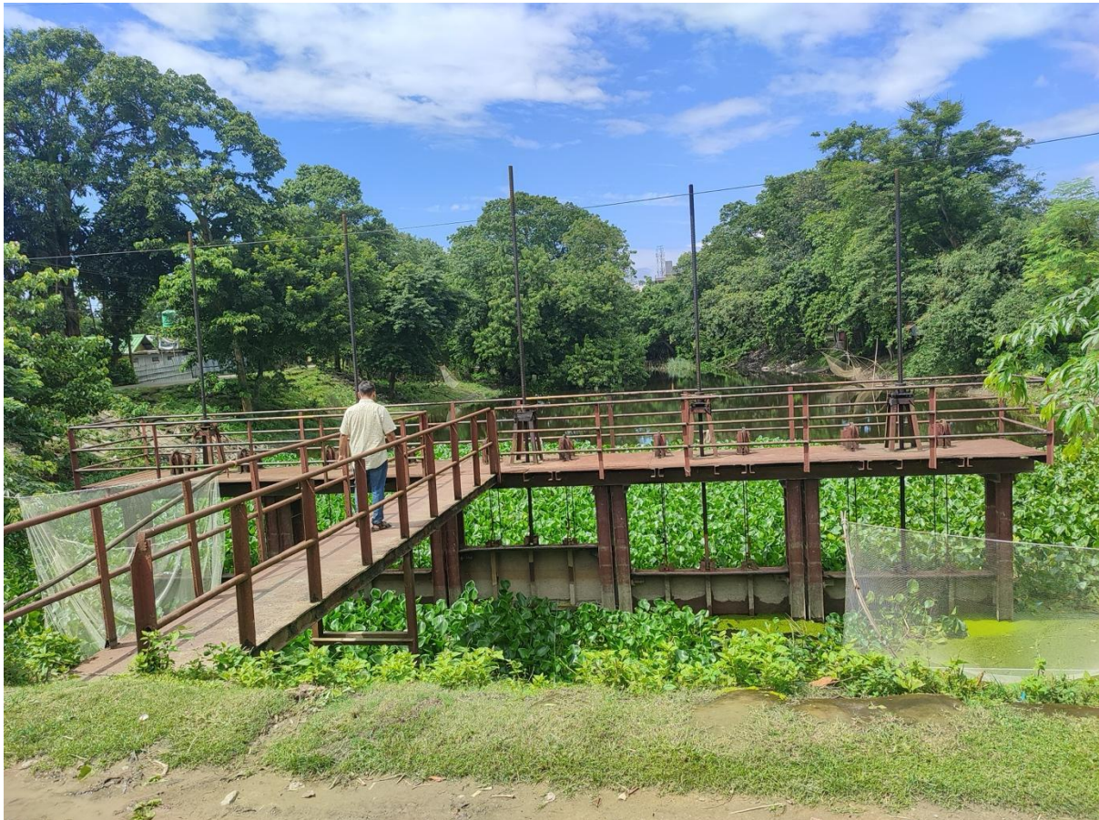
Photo 8: The Khanajan sluice gate in 2023. The gate of the sluice system remains closed during the rainy season which is also the breeding season of fish this blocks the movement of the fish from the Brahmaputra to the wetland (2023).
